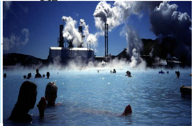
Fig. 3 Geothermal Power plant and Blue Lagoon
