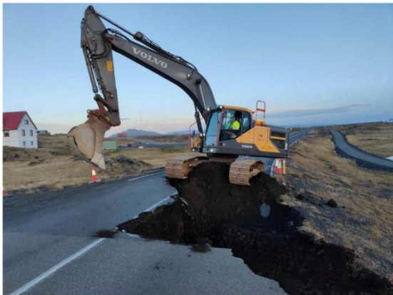
Streetworks continue after cracks emerged on a road due to volcanic activity near Grindavik, Iceland obtained by Reuters on November 14, 2023. Road Administration of Iceland via Facebook/ Handout via Reuters. TPX images of the day
